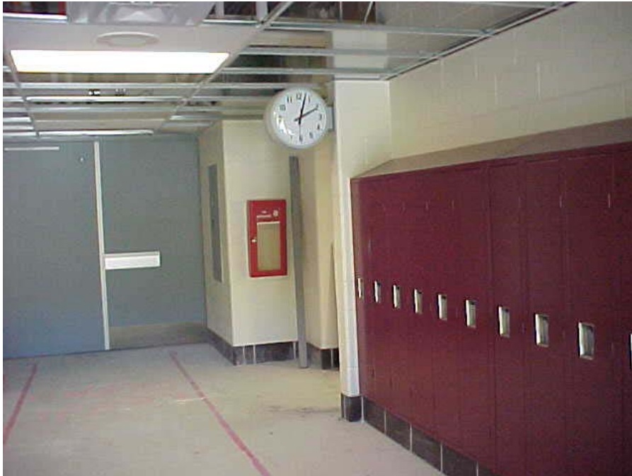
Corridor in Addition
