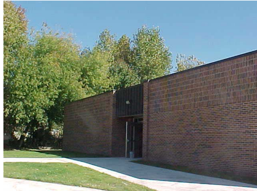
Exterior of Addition
