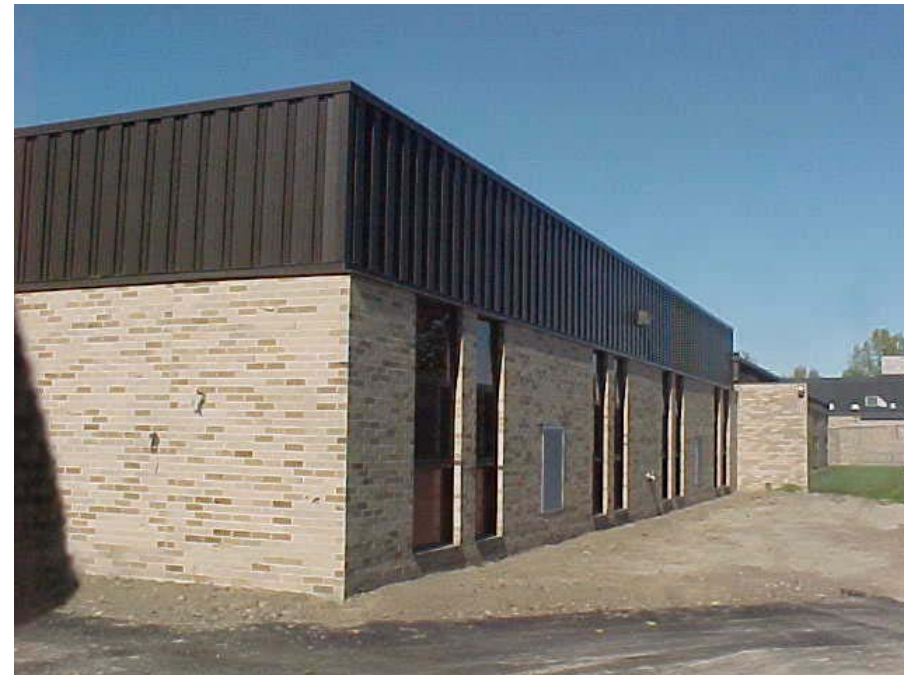
Exterior of Addition
